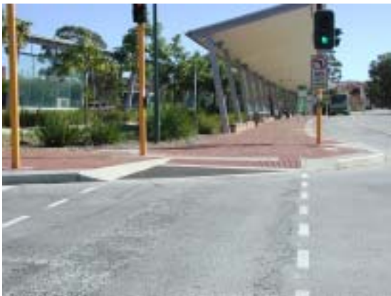
▪ Figure 8-1 Good Disabled Access Designed Ramp designed to current MRWA standards, Curtin University.
